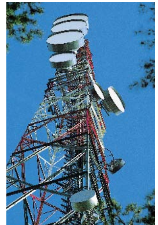
Getting ready to roll-out the billion pula Maitlamo project.
